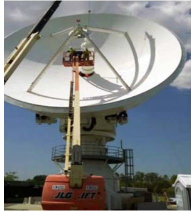
Installation of the W-2 antenna feed at WCDAS. Credit: Harris Corporation
